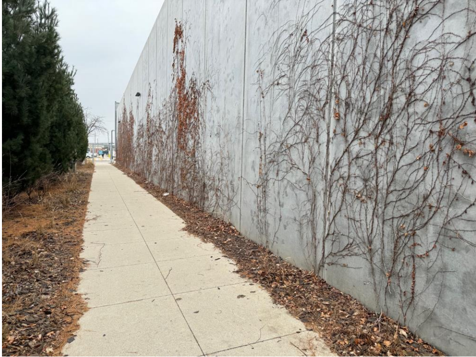
(View from midpoint in walking path looking towards 5th Ave)
